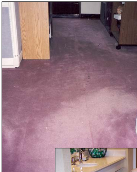
Traffic Lane Matting & Crushing
