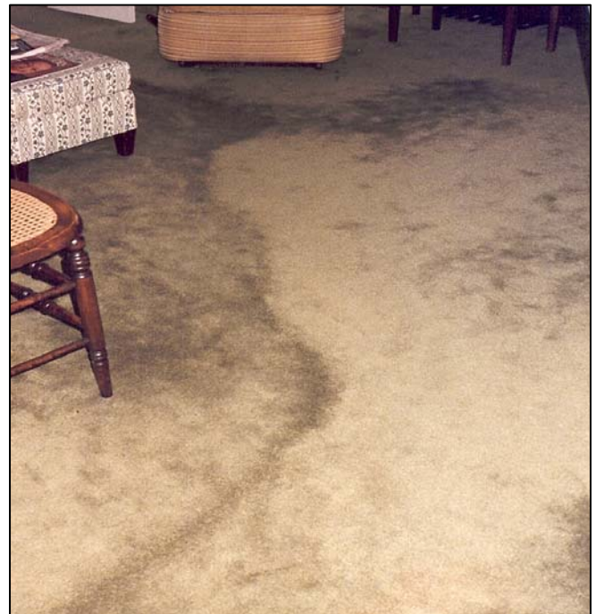
Watermarking & Pile Reversal - Residential
