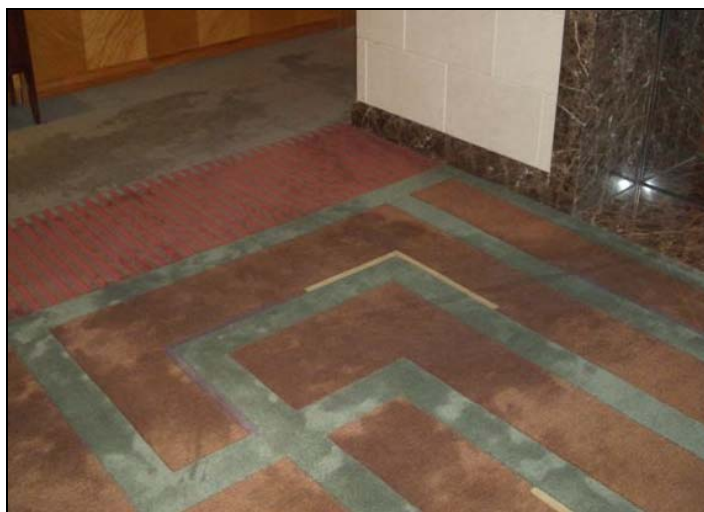
Pile Reversal & Shading – Elevator Lobby
